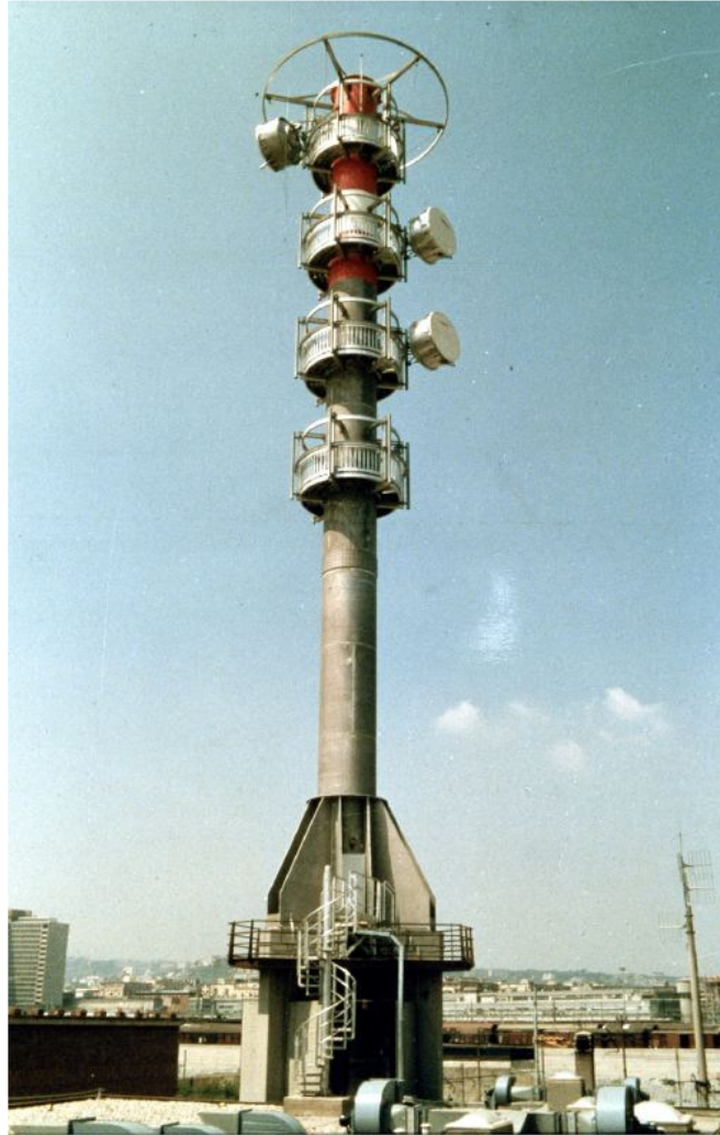
Figure 6: Tower for parabolic antennas.
